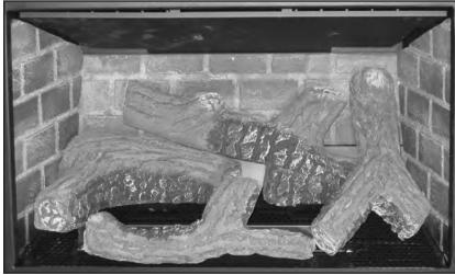
Figure 74. Fourth Stage Log Set Installation.
